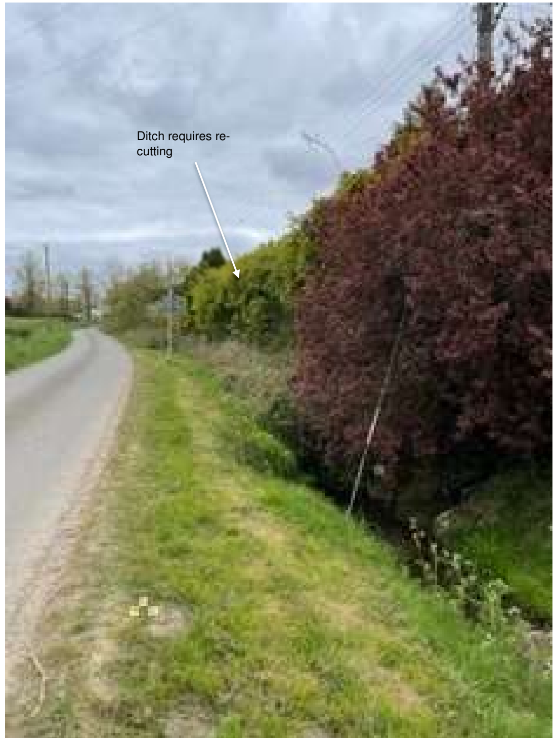
Point P13: Re-cutting and vegetation clearance required with care not to erode division between pond and adjacent ditch.
