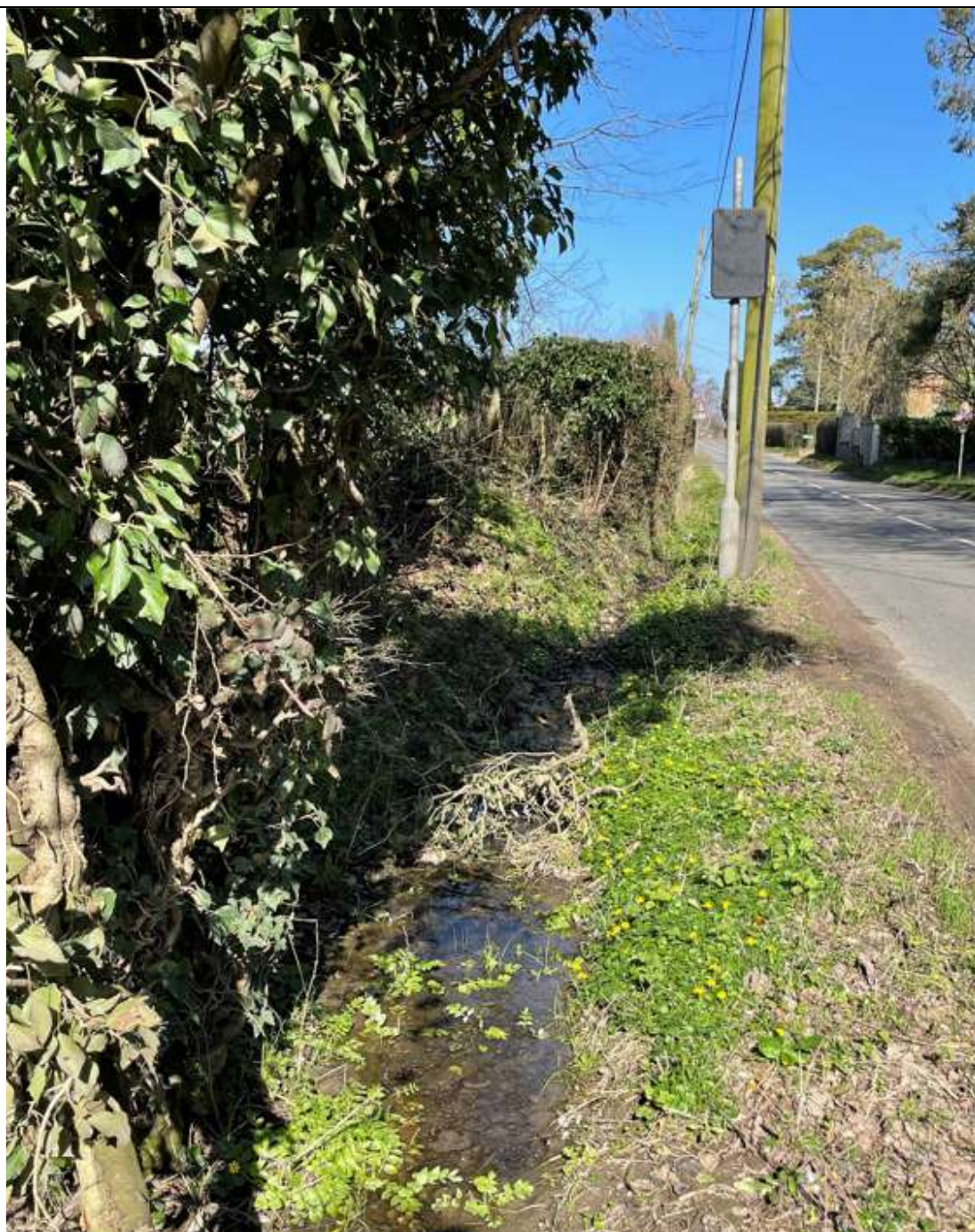
Point P2: Looking north from Hall Road up Church Road. Ditch network is silted up and requires clearance to improve flow towards the culvert under Church Road (ford in times of heavy rainfall).
